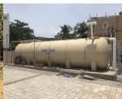
COMMERCIAL BUILDING (40KLD)
